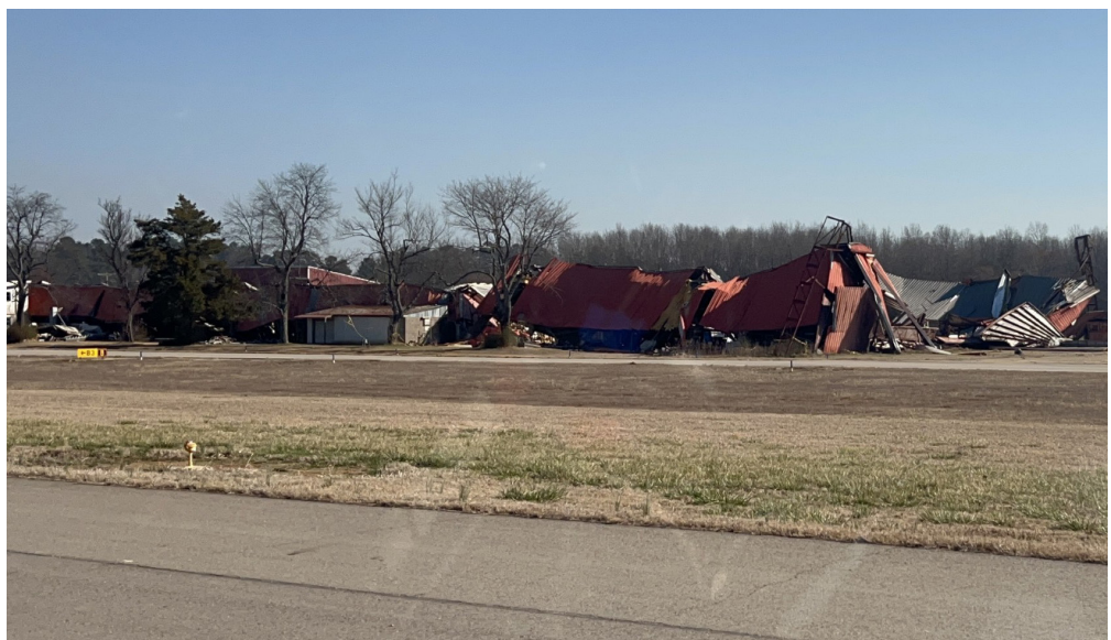
Another angle of the collapsed hangar.
