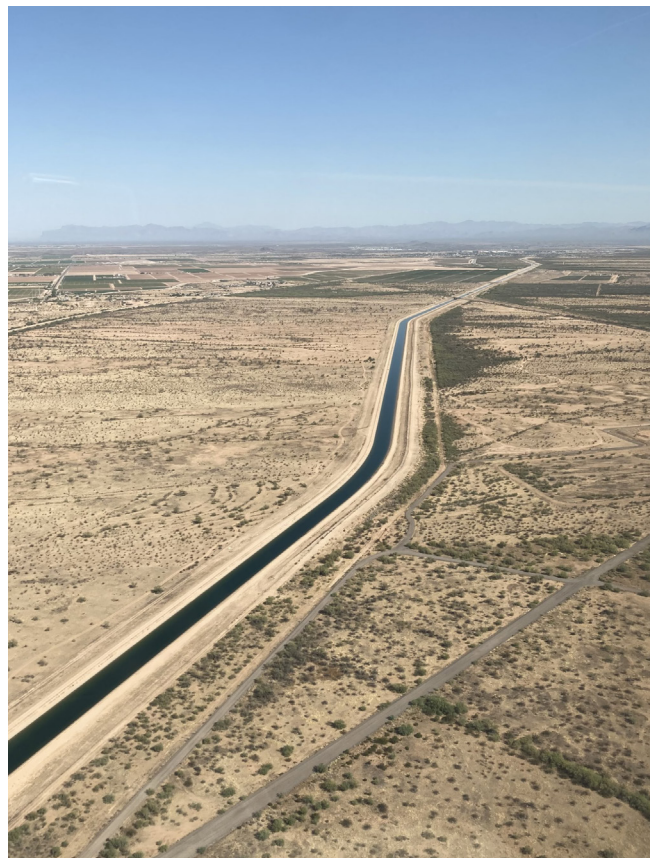
An aqueduct inbound
